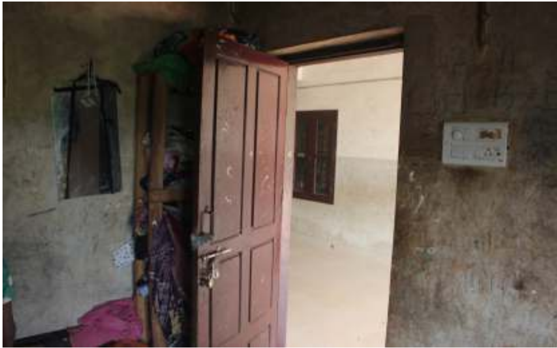
Picture 19. The main entrance door to the flat
