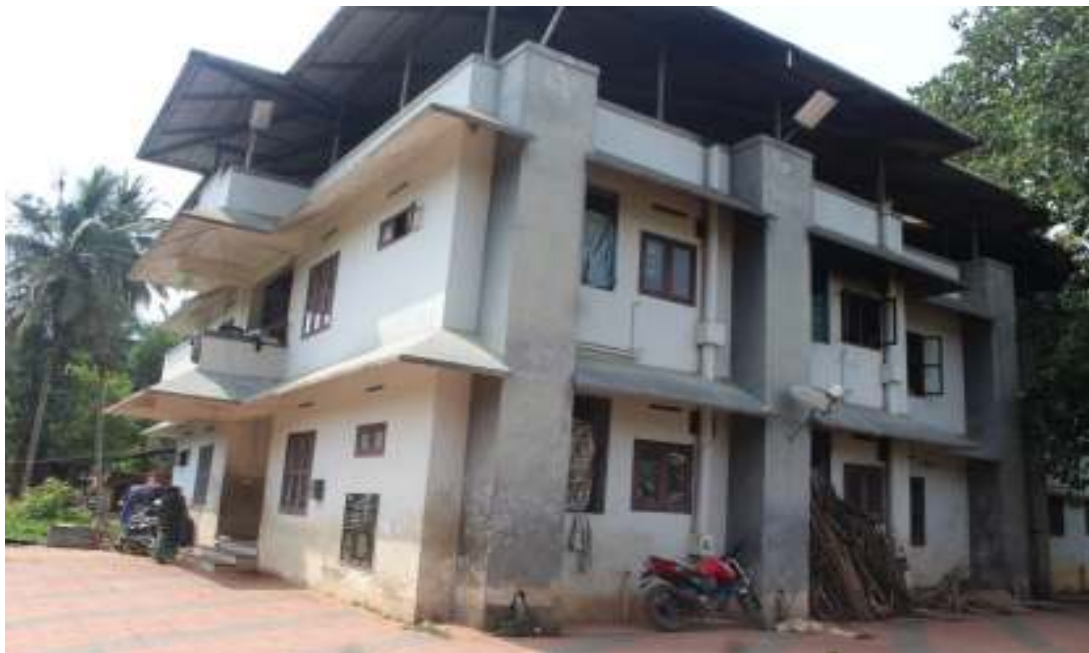
Picture 16. The first residential flat for the tribal communities, Kalpetta, Wayanad
