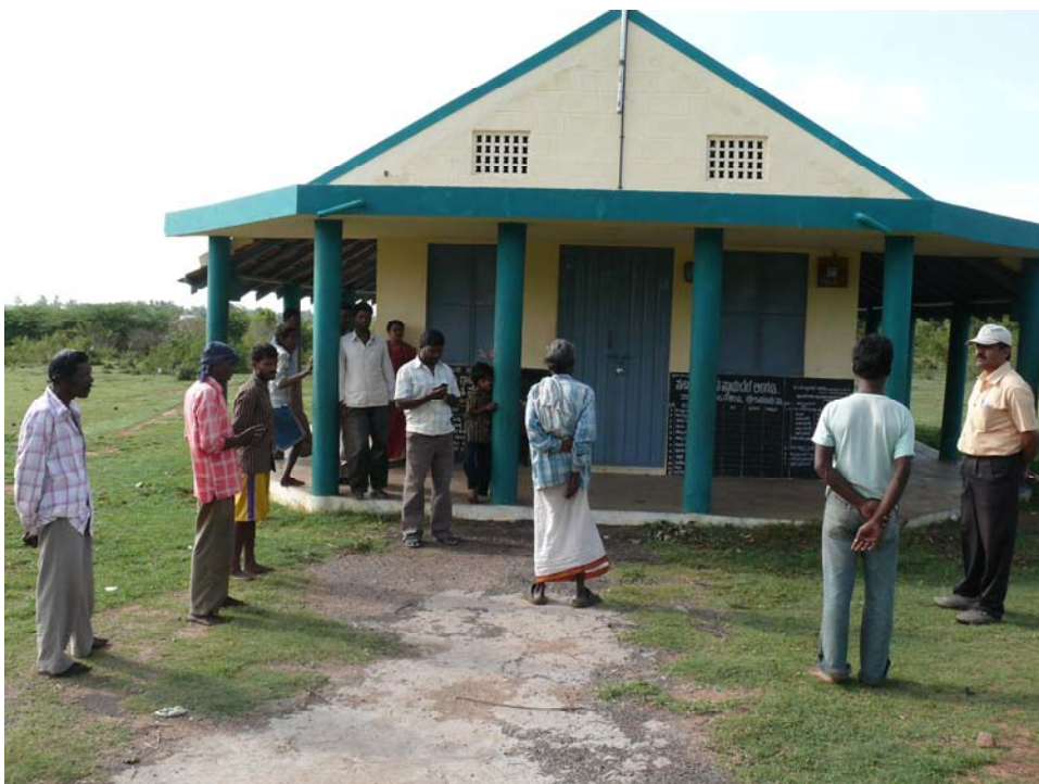
The re-constructed community hall at Nagapura Block IV
