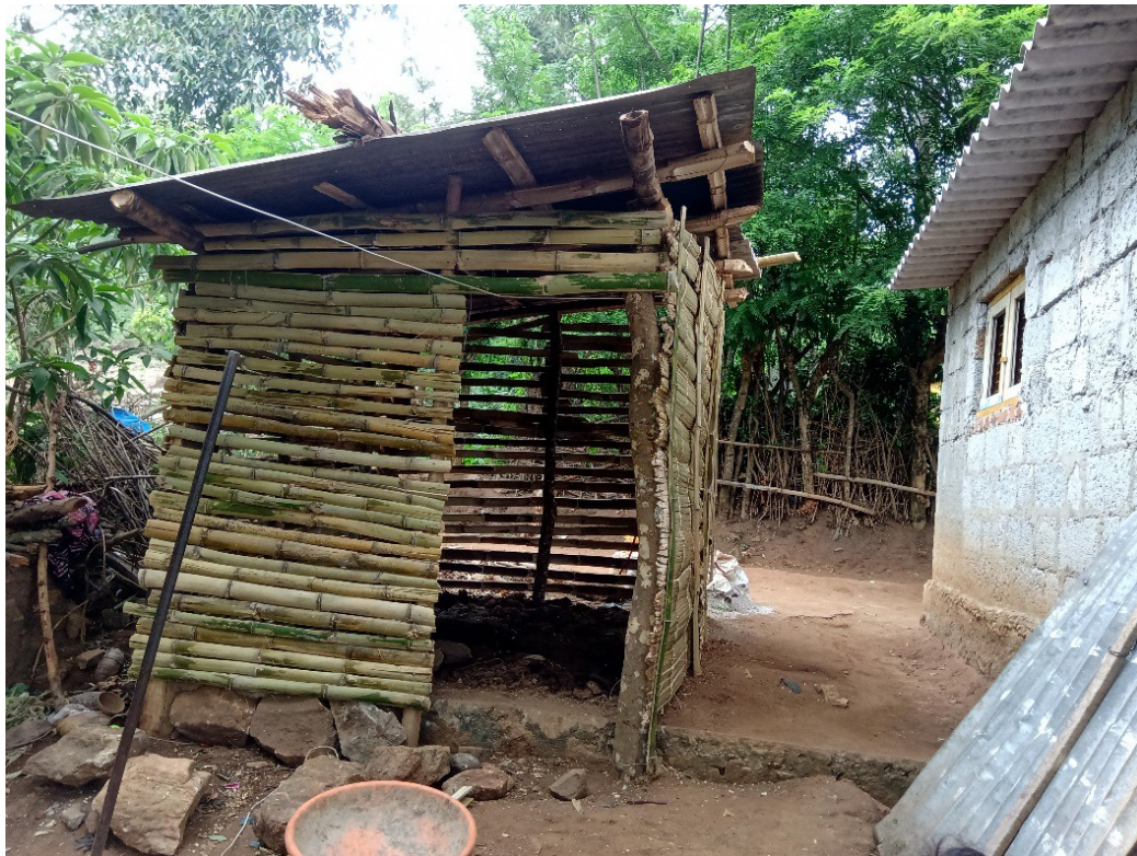
Figure 12 Bamboo kitchen built to cook with firewood
